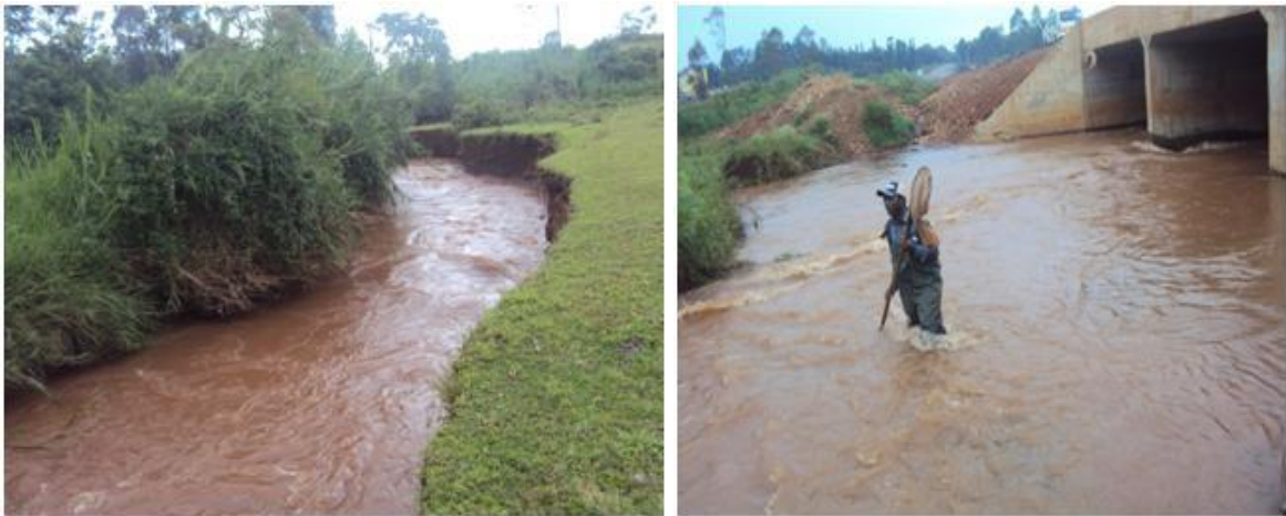
Plate 6. Kadongo Bridge sampling station
